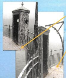
> Rains poured through the cracks from the upper deck into the "Cellar" below, preventing storage of supplies and further deteriorating the concrete structure.
