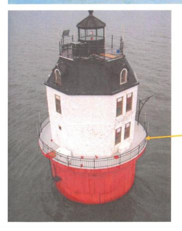
The new owners of the light wanted to stop the water leaks and also provide a safe walking surface on the upper deck. They contacted Acry-Tech and discussed the benefits of Soft Tread for creating a safe walkway around the light, even in inclement weather.
