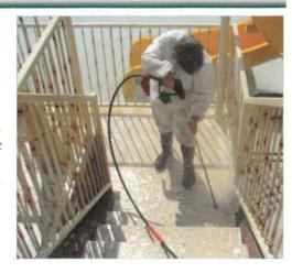
Rust Stains on the concrete and also on the fiberglass slides were treated with Acry-Tech's RustX Rust Stain Remover.
