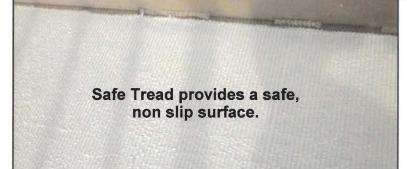
The maintenance personnel applied **Safe Tread** to the ramp surfaces and found that the **Safe Tread** filled the grooves and provided a safe footing for the students and teachers.
