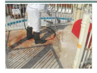
High pressure water blasting was required to remove years of built up, old blistered, peeling and delaminating coatings. A clean surface profile was achieved and will insure excellent adhesion for the *Safe Tread* application.
