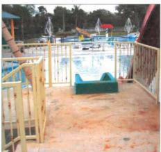
Previously applied non slip concrete toppings were stained, flaking and in need of serious attention. Acry-Tech Representatives visited the site and recommended the removal of all loose and flaking coatings using high pressure water blasting in order to create a clean, porous surface on which to apply *Soft Tread Anti-Slip Coating*. Rust stains also needed pre-treatment with *Acry-Tech RustX* rust stain remover.
