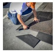
Transition ramps, with an ADA compliant slope are available for PopLock 1" thick tiles. These ramps come in two versions, with either male or female interlocking edges. Mitered corner kits are also available. Make sure that the correct ramp version, (male or female), is ordered. Do not trim the visible male interlocking tile edges in locations where transition ramps will be installed.
